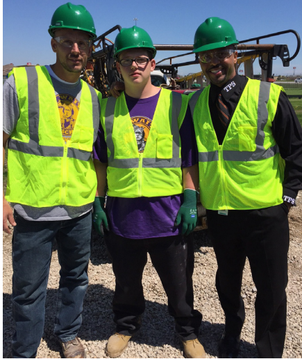
Toledo Schools Superintendent Romules Durant, right, tours a construction site with carpentry teacher Rob Materni, left, and student Boston Demecs.
